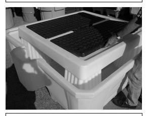
3.) Make sure grates are seated flat on center pedestal and pedestal seats firmly on all four towers.
